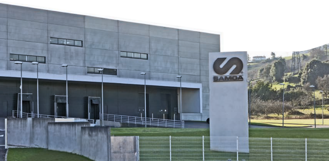
Headquarters Offices and Technical Centre in Gijón (Spain)
